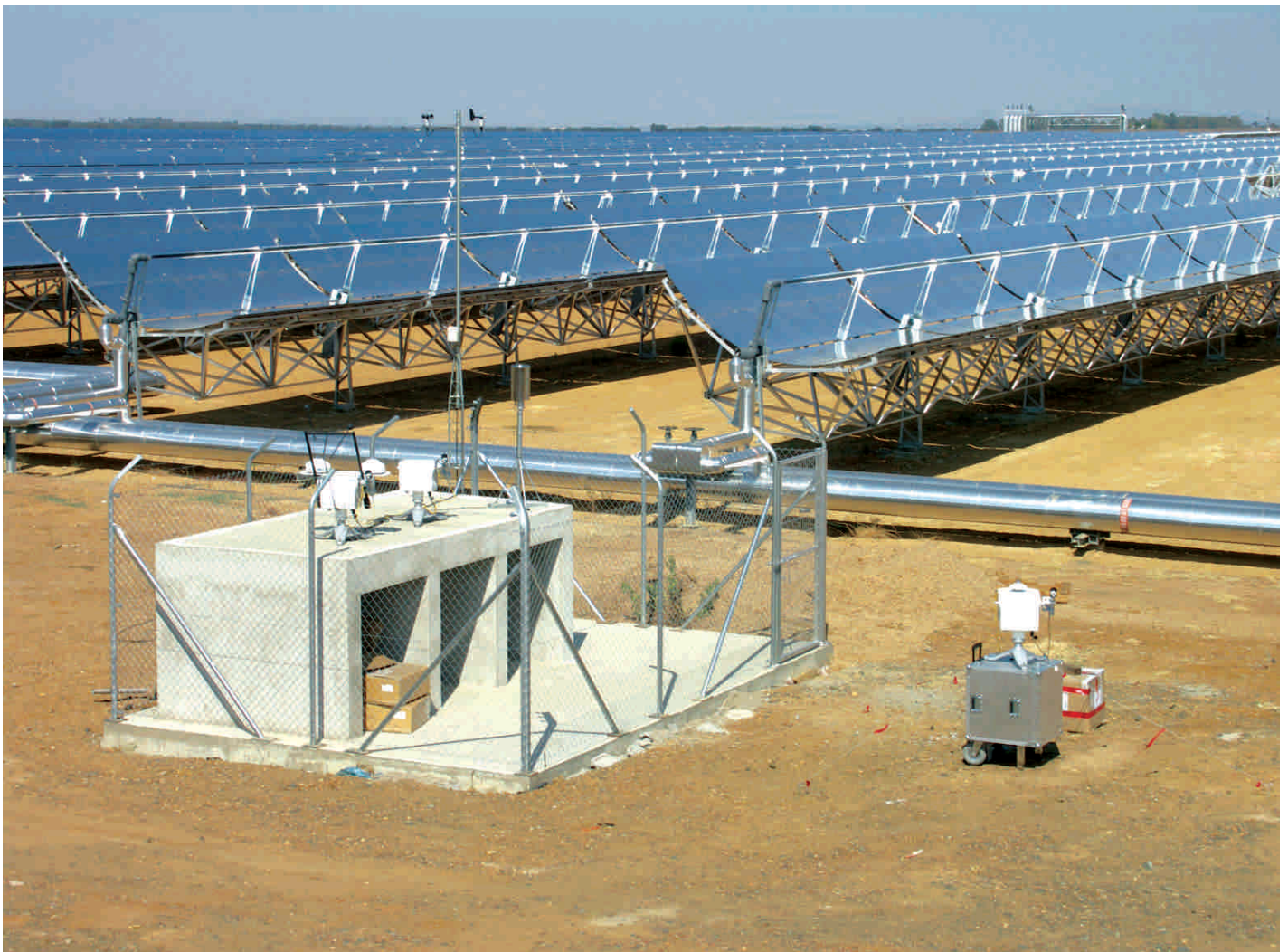
[Cener portable station at the Alvarado Plant of Acciona]
